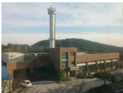
Figure 1. Picture of Power Plant Building
